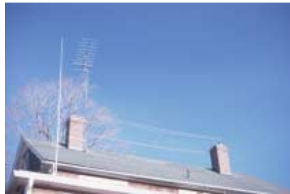
Third alternative: This photo shows a 15-meter version installed between two chimneys. It was built using wire and bamboo spreaders and with a rope arrangement to flip the antenna to favor one direction or the other. Plastic spacers were used along the wires to maintain the shape and spacing of each folded dipole. (AAIDO)
